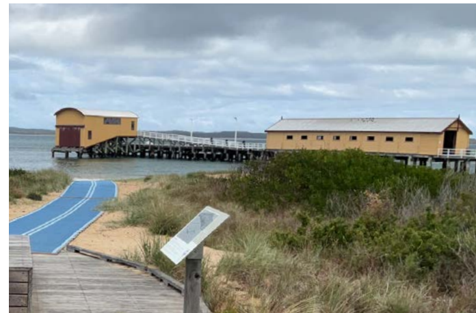
Queenscliff Pier - Queenscliff
